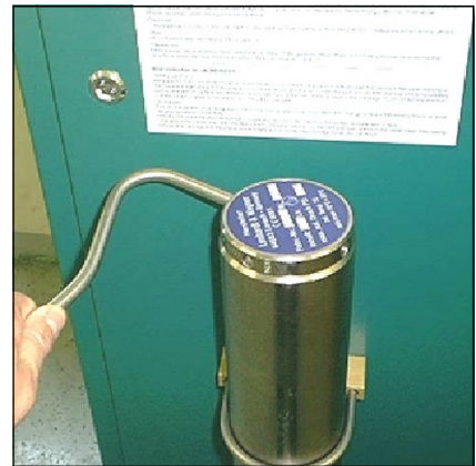
Fig. 1 - Unscrew the filter housing cover.
