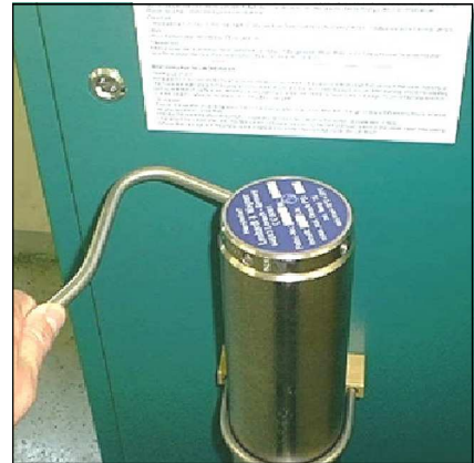
Fig. 1 - Unscrew the filter housing cover.
