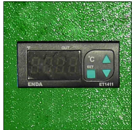
Oil Pressure Monitoring
