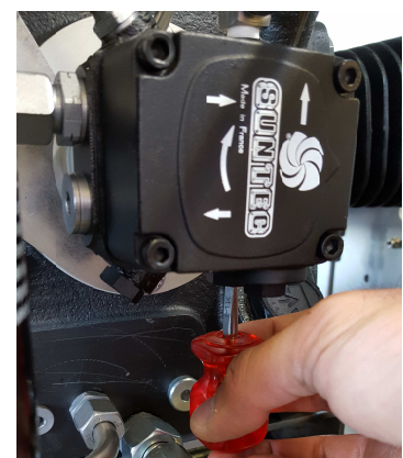
Adjusting the oil pressure
