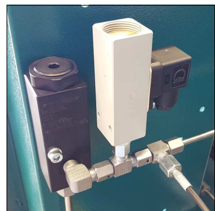
Pressure switch for start pressure
