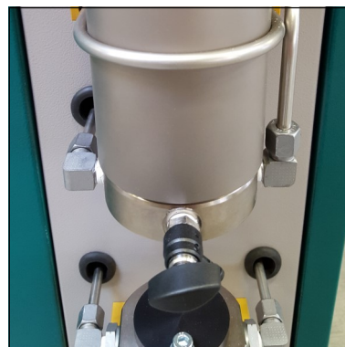
Fig. 3 - Loose pipe connections and nuts
